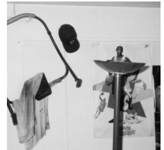
Where's the smoke alarm? Under the ball cap, next to the halogen lamp that started the fire in this dorm. The sprinkler head was able to do its job, even though it was being used to hold up a piece of gym equipment!
