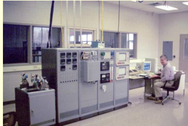
Mission Control Center at Composting Building
