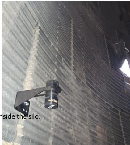
Figure 2 shows how one of the sensors is installed inside the silo.
