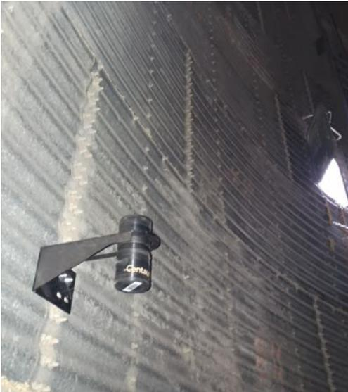
Figure 1: Example of wireless sensor installation inside a silo feeding the predictive algorithm with real-time data
